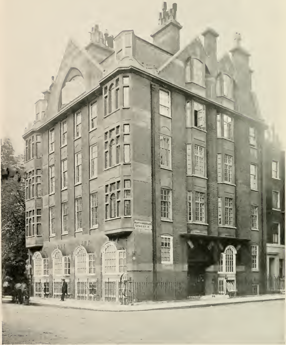
LUXBOROUGH HOUSE, NORTHUMBERLAND STREET AND PADDINGTON STREET, LONDON, W. THIS BLOCK OF FLATS HAS AN OPEN SITE WITH PUBLIC GARDENS IN FRONT AND AT THE SIDES. BUILT FOR TENANTS WITH MODERATE INCOMES, IT SHOWS THAT EXCELLENT DESIGN AND SOUND WORKMANSHIP CAN BE COMBINED WITH THE STRICTEST ECONOMY IN MATTERS OF EXPENSE. SEE THE PLAN ON PAGE 42
